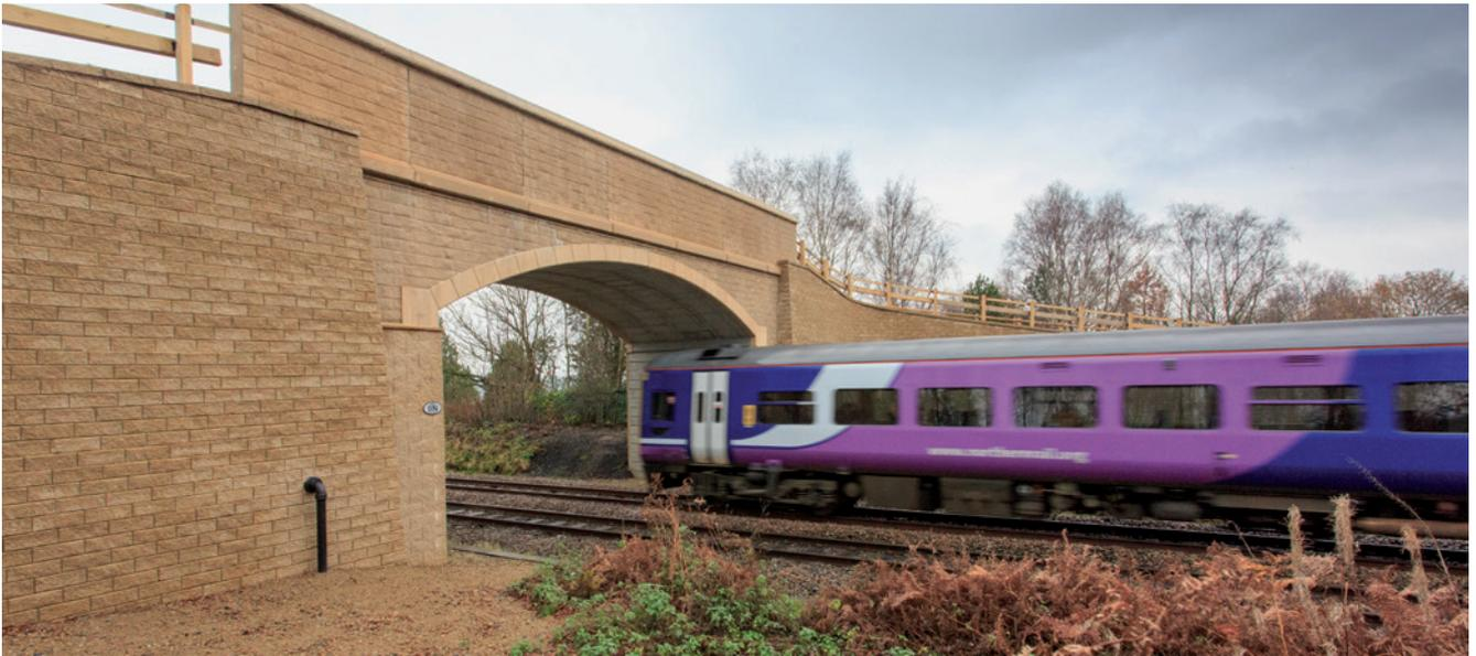
Our ethos of continuous product development and innovation has resulted in the company bringing to market a range of patented technologies such as the flexi arch bridge system, universal shaft linings and the vacuum-flush retention tank system. Since developing the flexi arch (pictured above) we have delivered more than sixty such structures across the UK and Ireland, and the system is also approved for Network Rail implementation.
