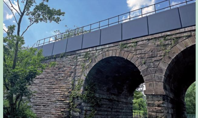
As part of the overall scheme to open a new station at Headbolt Lane, Kirkby, Merseyside and facilitate the laying of additional track Macrete Ireland Ltd supplied precast concrete robust kerbs pigmented black during the casting process to the reconstruction of UB56 on behalf of Buckingham Group Contracting & Network Rail.
