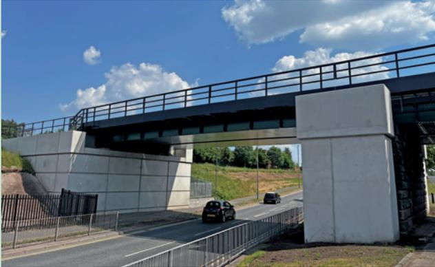
As part of the overall scheme to open a new station at Headbolt Lane, Kirkby, Merseyside and facilitate the laying of additional track Macrete Ireland Ltd supplied precast concrete abutment hollow blocks, wing walls, coping walls and cill beams to the reconstruction of UB55 on behalf of Buckingham Group Contracting & Network Rail.
