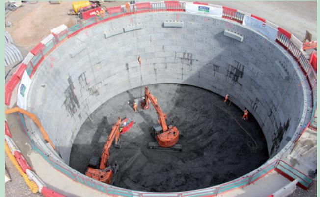
Macrete Ireland Ltd supplied 3.05m, 5.00, 6.00m & 25.00m shaft linings and corresponding cover slabs to the upgrade of the sewer and drainage system around Stroud Gloucestershire. The aim of this scheme is to provide a reliable sewer network and create more storage capacity in times of flood. By doing so, the local river health will also benefit. Materials were supplied to Galliford try on behalf of Severn Trent Water.
