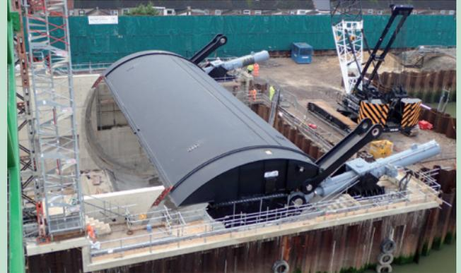
Macrete supplied 24nr precast concrete flood defence units for incorporation into the tidal barrier works. The units were in the shape of an inverted arch and would provide the base for the movable steel tidal barrier once installed.
