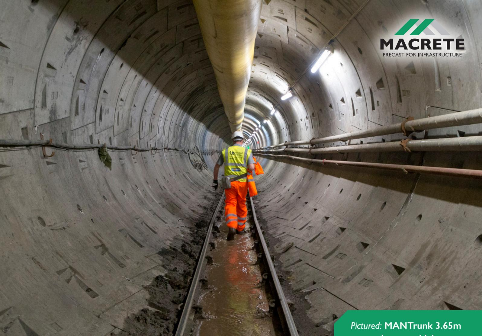
*Pictured: MANTrunk 3.65m tapered trapezoidal tunnel linings*
