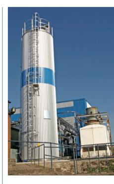
Above: Silo installation including cooler for chilling of rusk for well known brand of sausage manufacturer.
