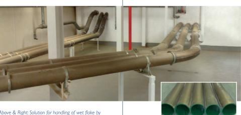
Above & Right: Solution for handling of wet flake by Teflon coating of pneumatic conveying pipework and components.
