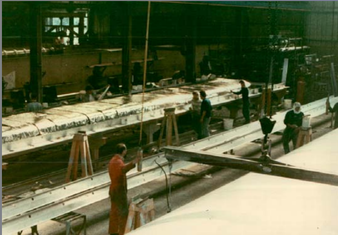
Roof assembly under construction.
