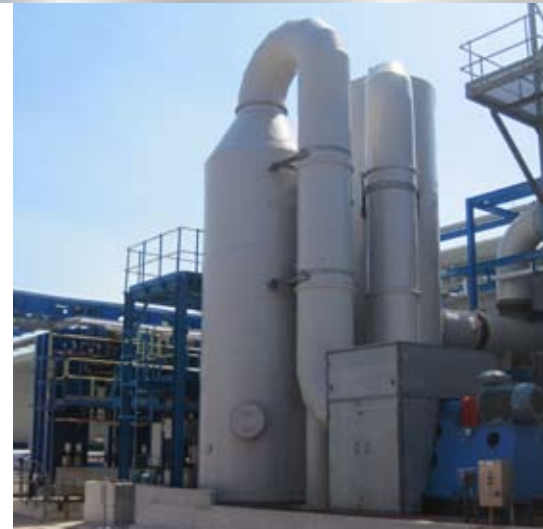
Waste gas treatment in manufacture of alumina based fibre, UK
