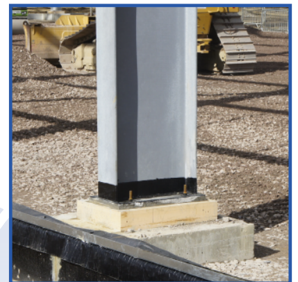
Column Base Thermal Break
