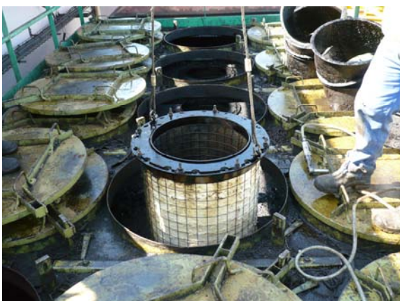
Xtra-Pure Inner Bed Candle Filter being lifted through removable roof plates
