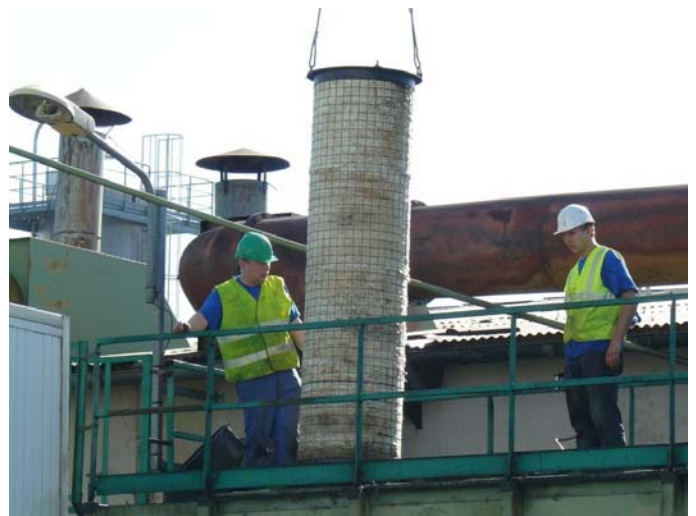
HT2 Candle Filter being lifted for inspection
