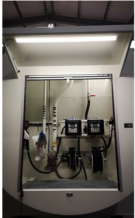
FULL HEIGHT CABINET HOUSING DUAL DISPENSING SYSTEMS
