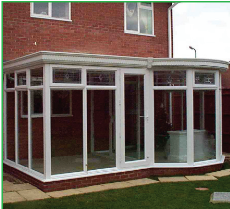
Flexi roof & Colwall combined
