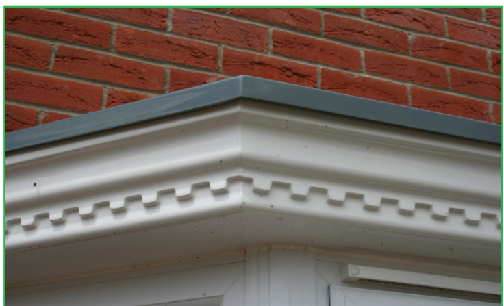
Victorian fascia close up
