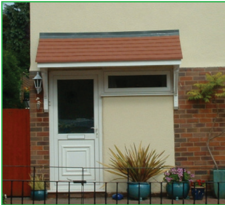
Westbury covering door & side window
