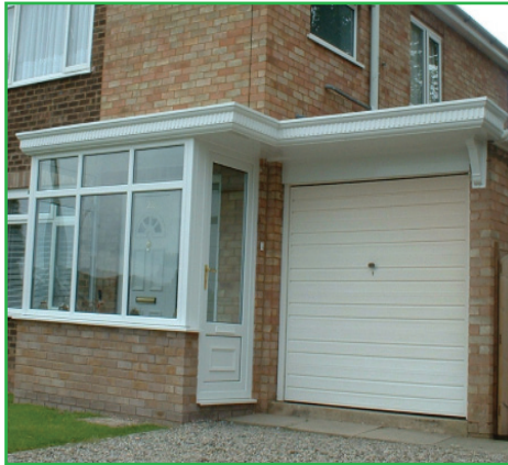
Flexi porch extended fascia over garage
