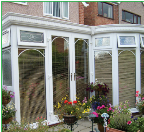
Flexi roof & Colwall combined
