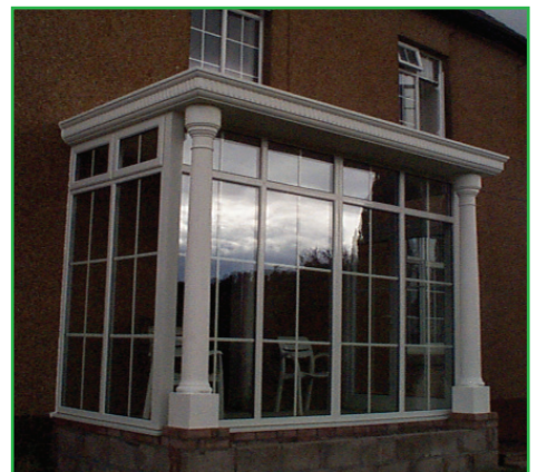
Flexi roof combined smooth columns
