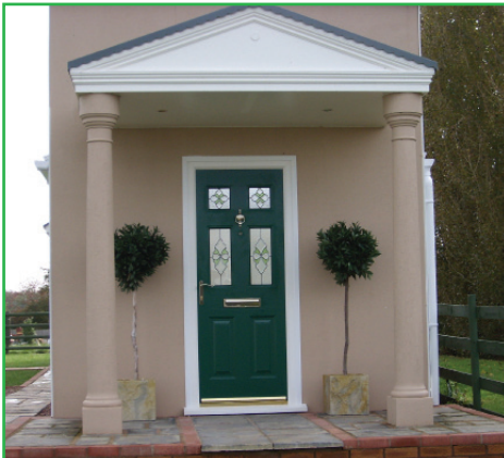
Alderbury & Smooth columns painted
