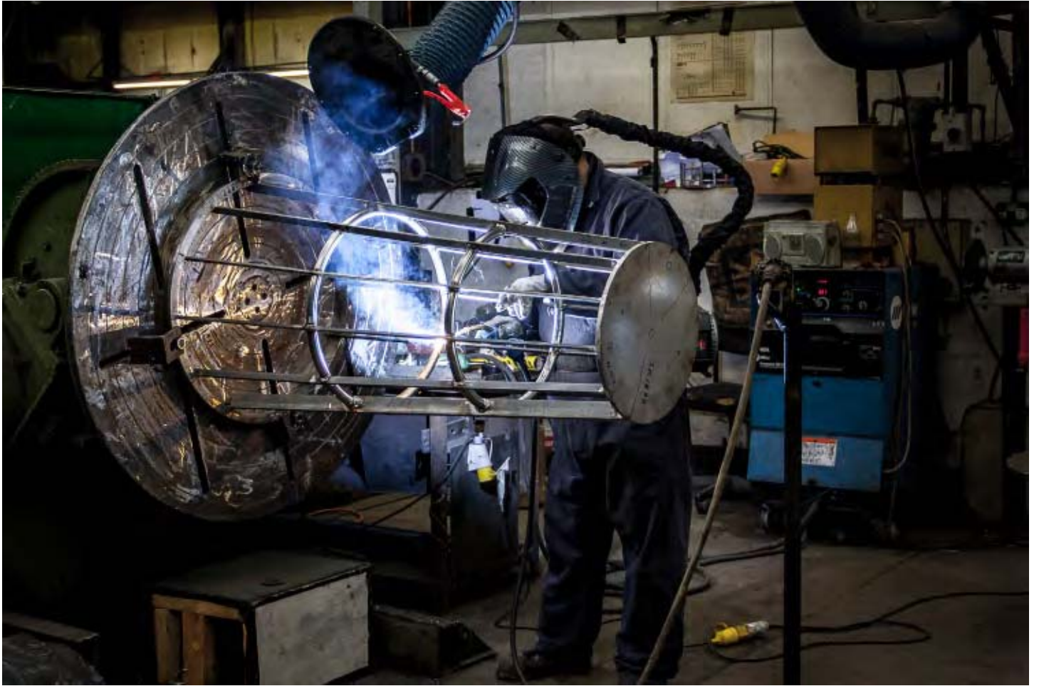
Best Practice: Welding of the internal element frame
