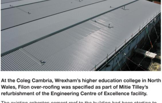
The existing asbestos cement roof to the building had been starting to fail and the resulting water ingress was causing damage to the roof structure and putting high value machinery inside the building at risk.
