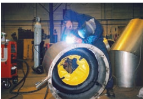
Speedy Purge used to weld a stainless steel elbow.
