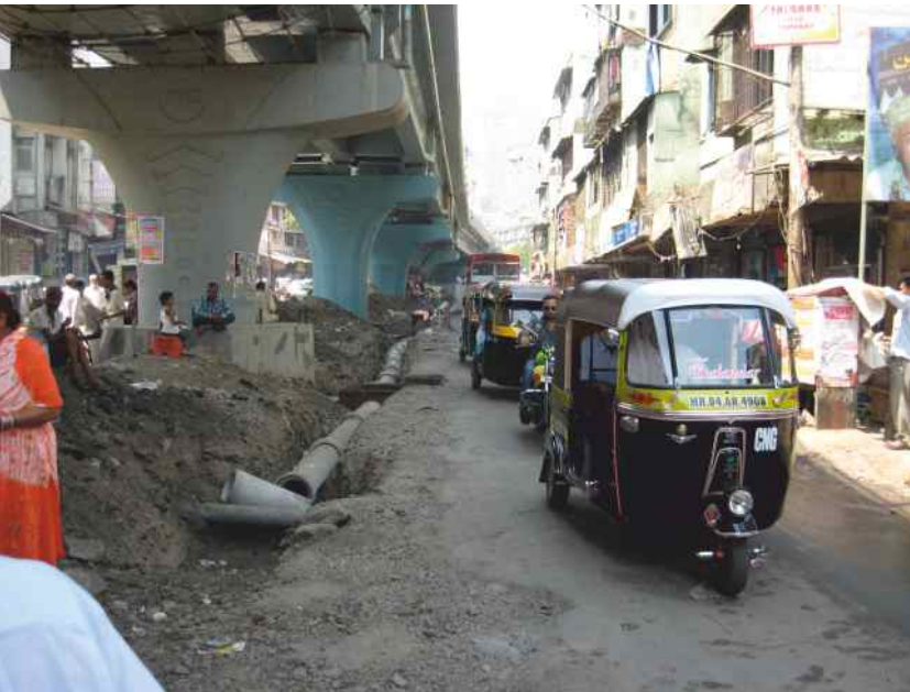
Above: Open cut installation Opposite: Sorry for the inconvenience
