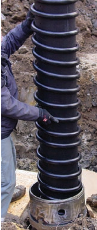
Installation by using a hollow auger drill
