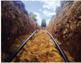
Standard PE100 – Sand Required
