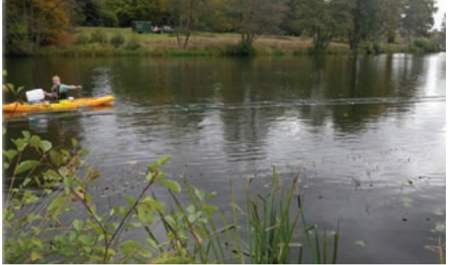
Our Lake Weights being deployed (once the pipe is filled with Glycol, the pipe will sink)
