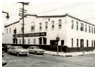
Warehouse and shipping building at 2nd and Columbia in Philadelphia
