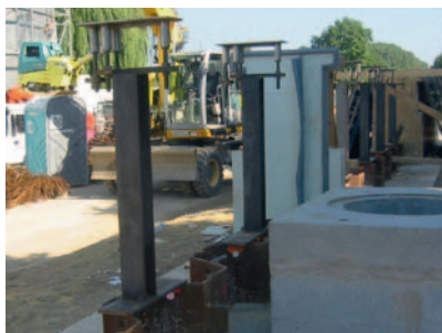
Assembly on sheet piling with cantilever for height compensation
