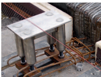
Assembly on subbase
