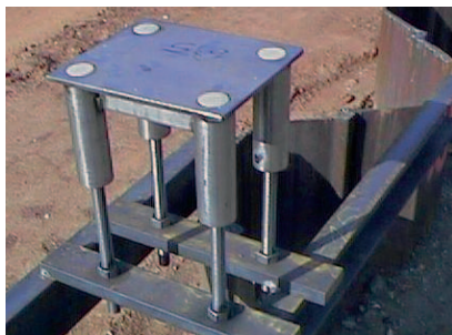
Assembly on sheet piling
