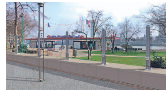
Assembly of center posts
