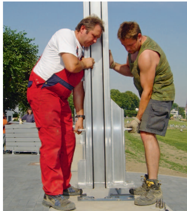
Two men carry a centre support post for flood height 2.10 m
