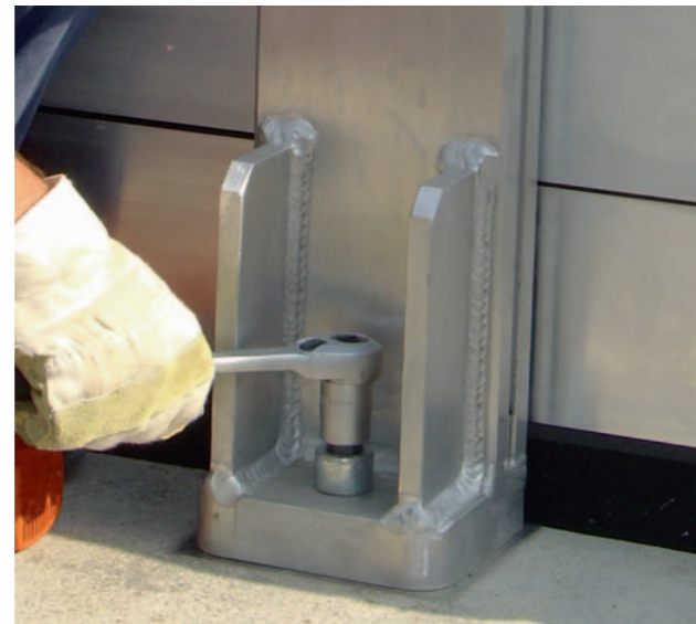
Bolts from the centre support foot and pressing tool
