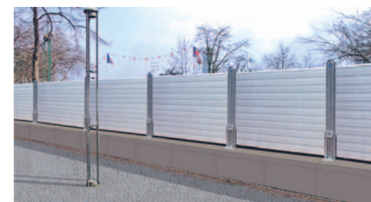
Complete flood protection wall
