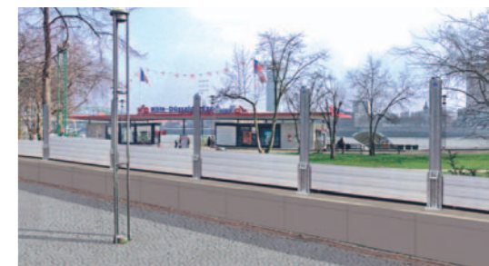
Center posts with dam beams
