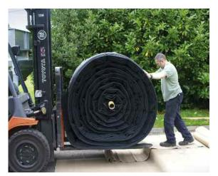
A 1.00mm Greenseal Geomembrane 26m x 53m being prepared for use as a dirty water lagoon at a dairy farm in Taunton.
