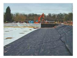
Greenseal Geomembrane being installed for a reed bed (Rockwood).
