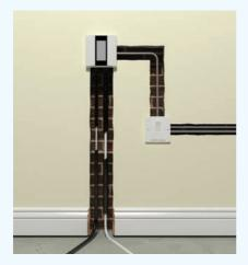
Before starting the installation you should make provision for the electrical connections, for smaller areas this may be possible by means of a switched fused spur with an appropriately sized fuse or a combined RCD spur from an existing circuit - **see above**. However for larger areas a dedicated circuit from the consumer unit will be required - you should always consult with your electrician concerning your specific requirements.
