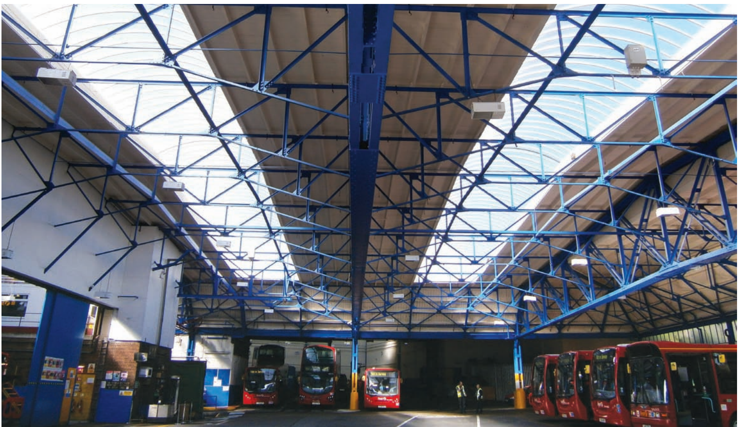
The Finesse system comprises multiwall polycarbonate glazing with steel channels for ease of installation and high strength.
