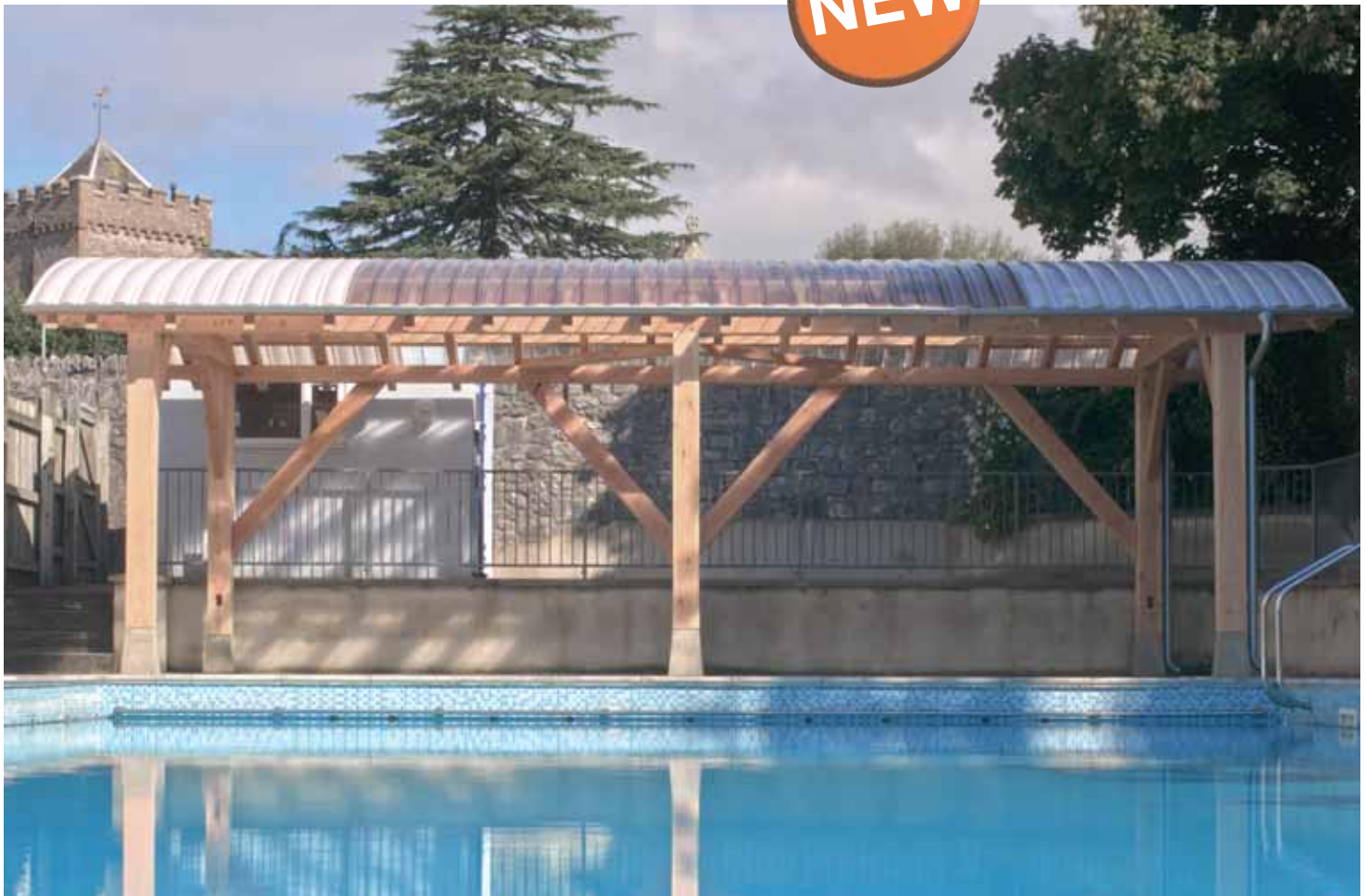
Fastlock panels are mounted to Timber Design's Blau Shelter structure to form the canopy at Chudleigh's Community Swimming Pool, Devon
