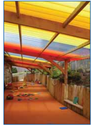
Canopy at Willesborough School, Kent, by Orchard Priory Ltd.
