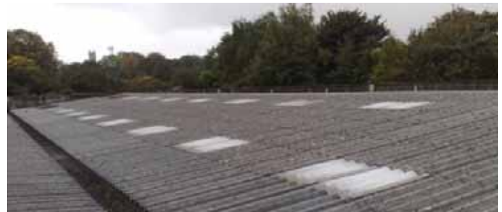
Fragile acrylic rooflights at HSBC's Manchester facility required urgent replacement
