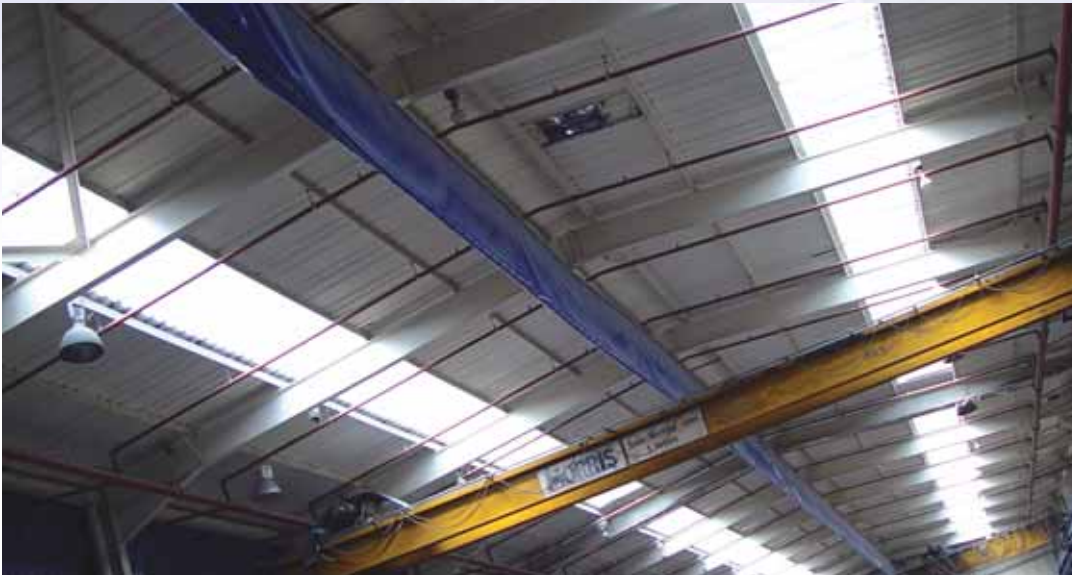
New rooflights in the FILON factory are making a contribution to energy saving
