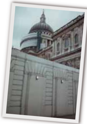
FILON GRP site cladding near St. Paul's Cathedral, c.2000
