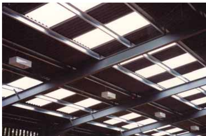
Natural light saves energy and reduces carbon emissions. Larger rooflight areas provide a cost-effective route to compliance with the Building Regulations
