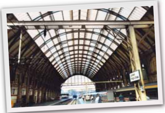
London's Kings Cross Station in the eighties. The canopy features FILON rooflights
