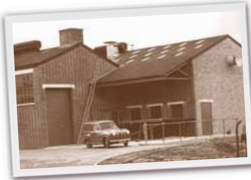
The boiler house and resin deck at FILON's original factory at Streetly, November 1957
