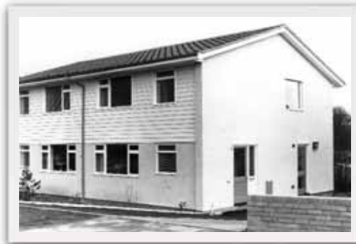
FILON GRP cladding on domestic properties, mid 1960s
