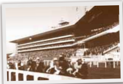
Royal Ascot, early 1960s. FILON GRP roof underlining used on the new grandstand
