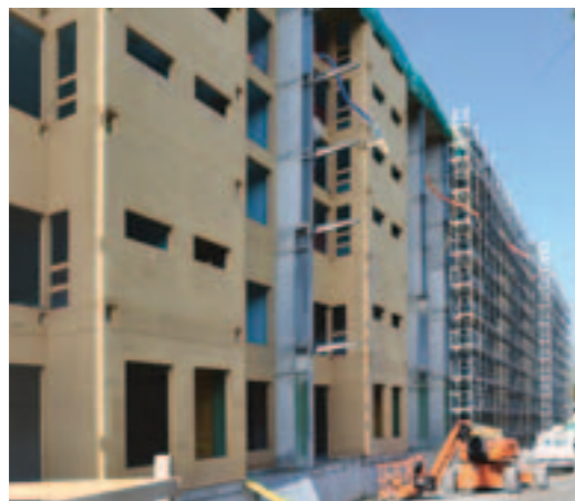
Hybrid construction with 60 mm DIFFUTHERM in Fribourg, Swiss
