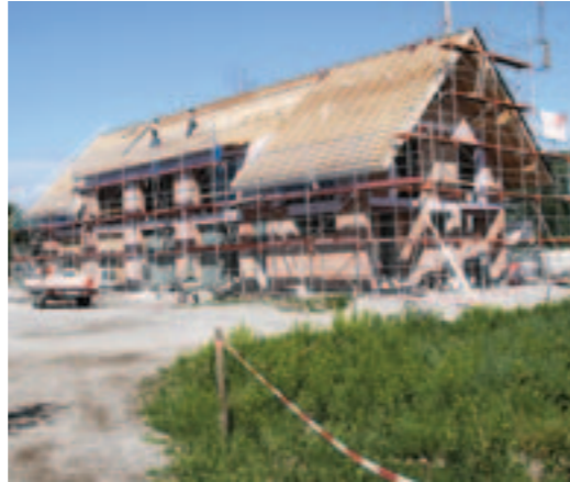
Typical over-rafter insulation – simply applied full-surface insulation in Legau, Germany.
