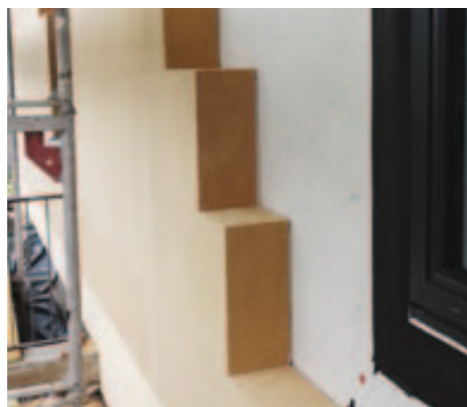
PAVAWALL-BLOC can be mounted directly to stone- or timber substructures.
