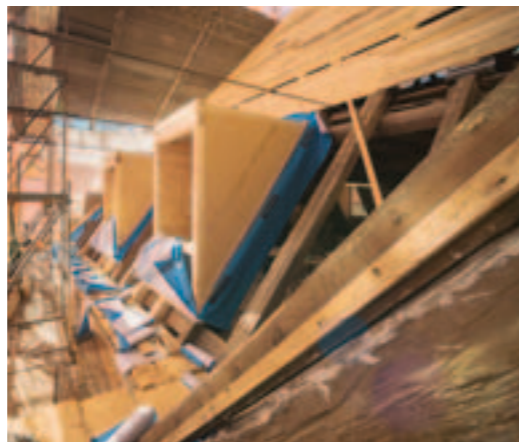
The PAVATEX insulation system is particularly effective for the renovation of protected historical buildings, such as this charterhouse in Freiburg, Germany.
