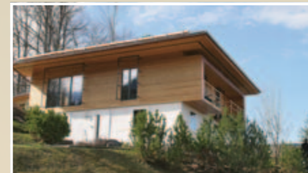
This building was modernised and given a timber façade in Bad Dürrenberg in Austria. PAVATEX woodfibre insulation was used for energy-efficient insulation of the building fabric.
