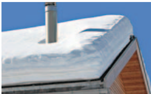
An optimally insulated roof has the same temperature as the surroundings so that the snow remains on the roof.
