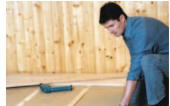
PAVATHERM-PROFIL is a compression-resistant, soundproof woodfibre insulation board for floor constructions.
