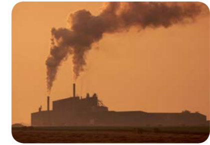
Industries, HVAC & Marine
