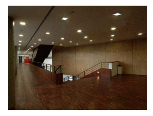
Square recessed luminaires made from aluminium frame - anodised
