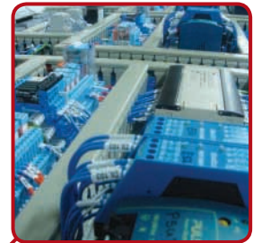
Control Panel Assembly
