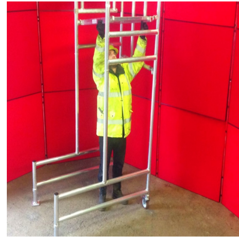
2) FIT PLATFORM AT CORRECT HEIGHT
