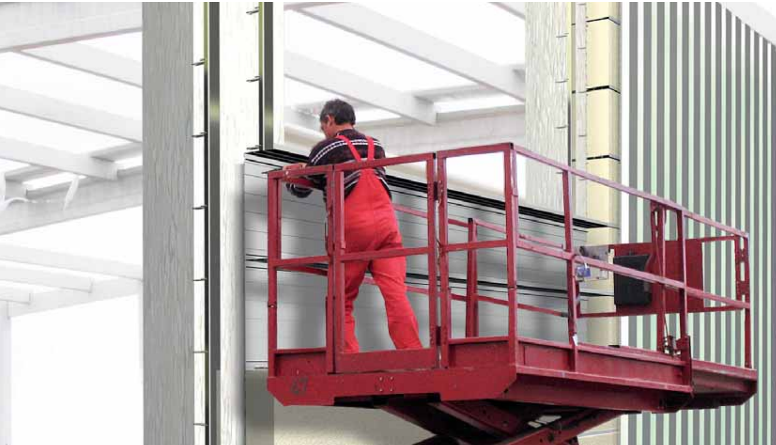
Installation of a multi-layer insulated profiled metal sheet wall.
