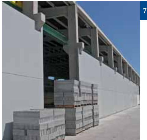
Industrial building quickly installed using large concrete components, Anchors Channels, T-bolts and brackets
