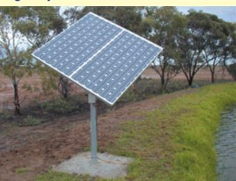
A GPS (Global Positioning Satellite) sensor built into the controller provides precise latitude, longitude and time. This is all that the controller needs to calculate the exact position of the sun and correctly position the solar array.
