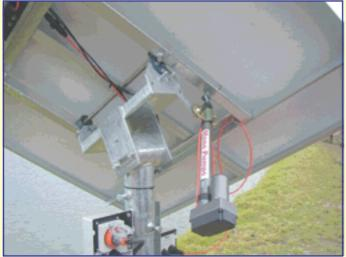
The Mono GPS Tracker (patent applied for) will ensure that your solar modules are always facing the sun. The GPS Tracker overcomes the problems that are traditionally associated with refrigerant gas and light sensor trackers to ensure 100% tracking accuracy in all conditions.
