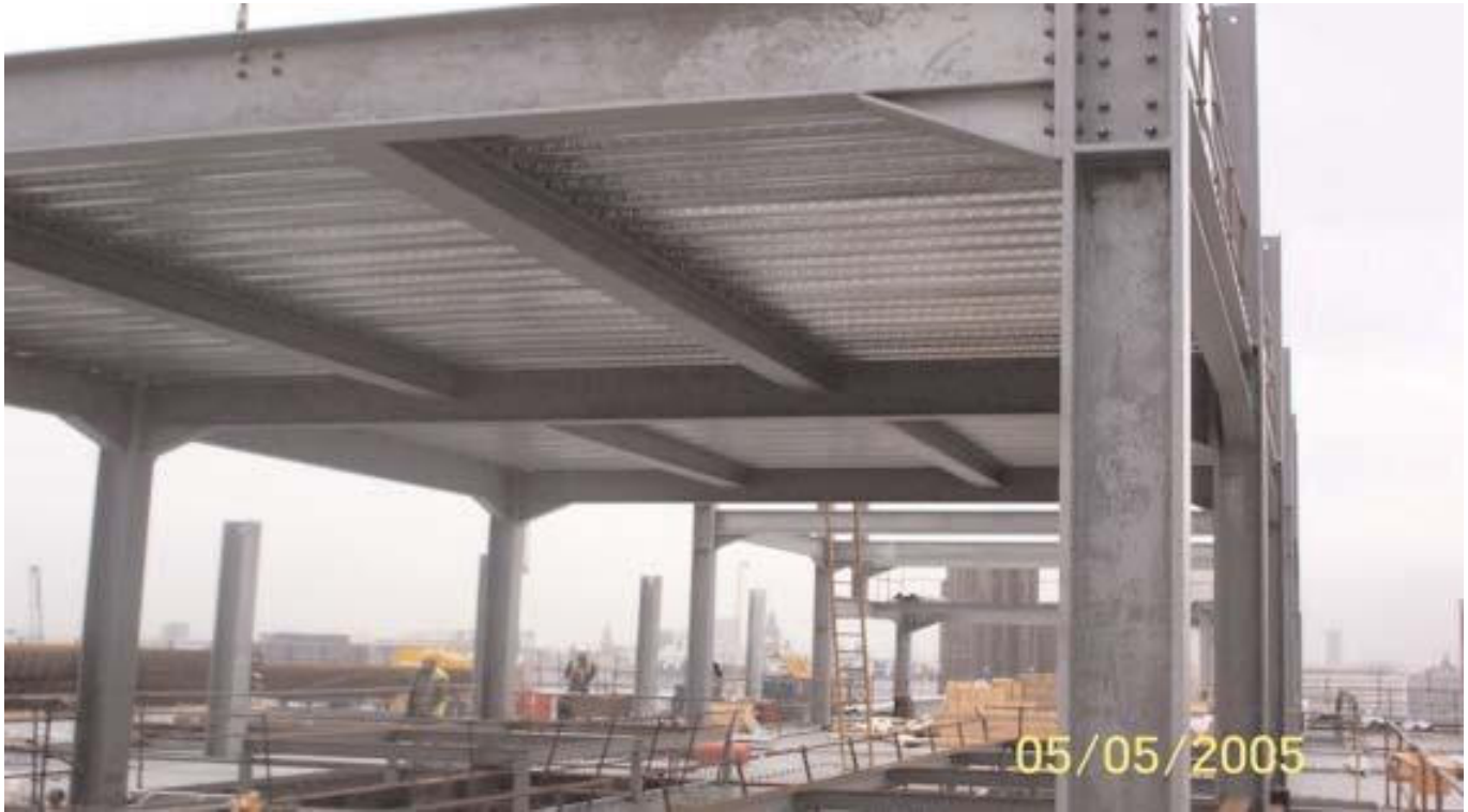
Lift machine room structural steelwork
