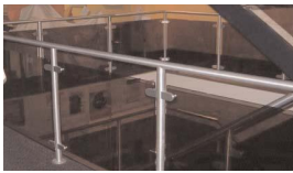
Supply & Fit Handrail Page 23
