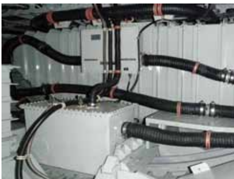
Above: rear bay tank installation
