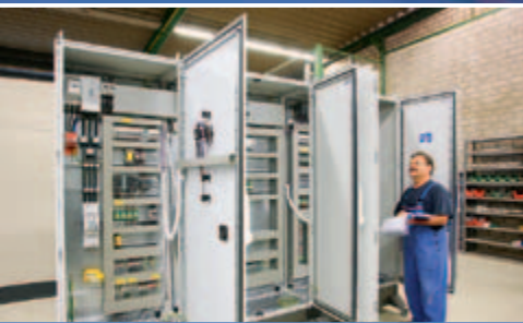
Control panel construction
