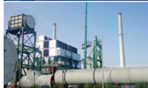
Erection of plant
