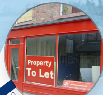
Empty Property And Asset Protection
