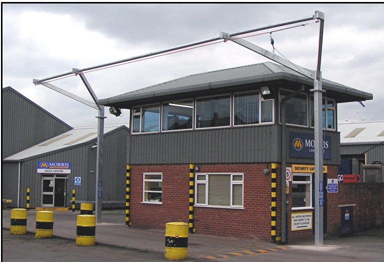
The photograph on the left shows a typical example of the installation of a Line type Fall Arrest system used, in this application, to provide safe access to the top of Road Tankers.
