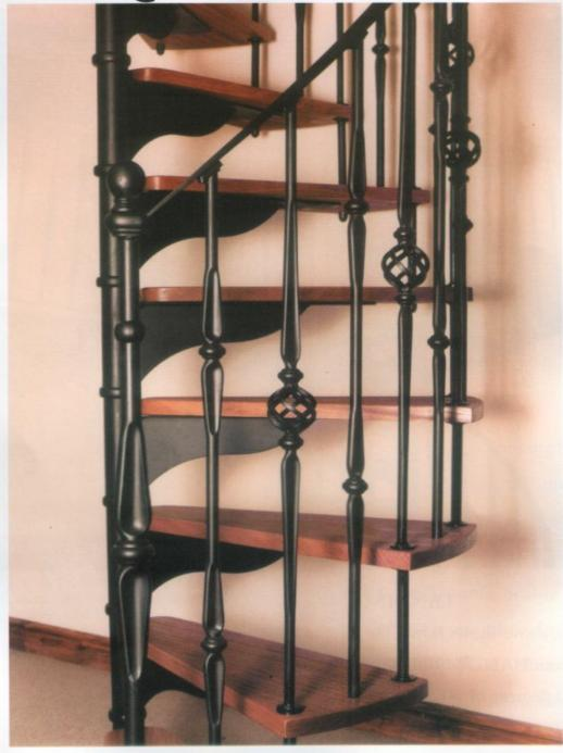
This close-up picture enhances the SUPERB QUALITY of the Balusters. The Stair incorporates the Scalop Newell Post (PC630) complete with Cast Finial for the Handrail fixing. Stairs are available with bottom Handrail SCROLLED as to the front cover of the TRADITION Brochure.
