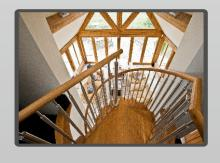
Because we use an open faced tread design, the stair allows plenty of light to pass through. Together with the stainless steel core and balusters, this gives a clean and bright appearance.
