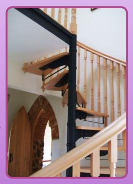
This practical spiral staircase is ideal for Barn conversions or serving a Mezzanine or balcony. This image shows the solid wood beech treads with the balusters attached. This stair has been fitted with a metal riser bar to adhere to the 100mm gap rule and is generally used when small children are using the staircase
