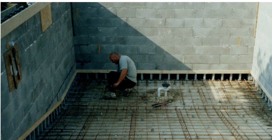
Introduce steelwork to floor; tied to wall steelwork to engineer's specifications.
