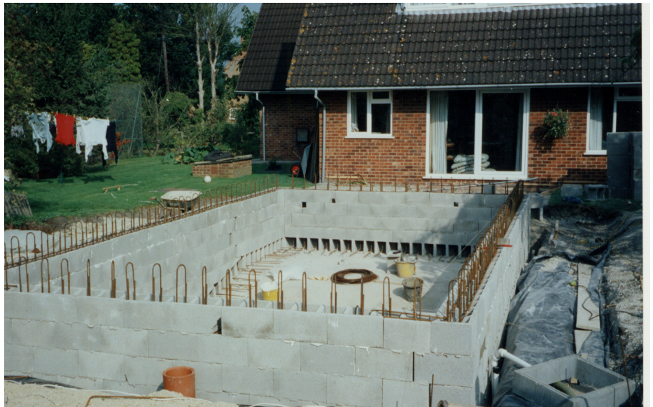
Last row of vertical steel with hoops to engineering specification.
