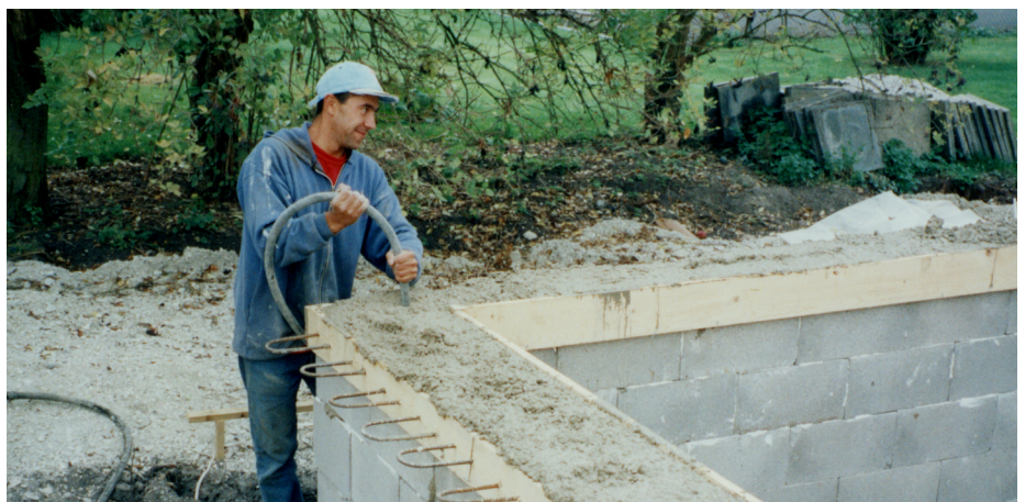
Level floor. All concrete must be vibrated.
