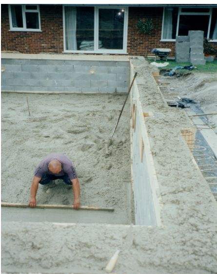
Level floor. All concrete must be vibrated.
