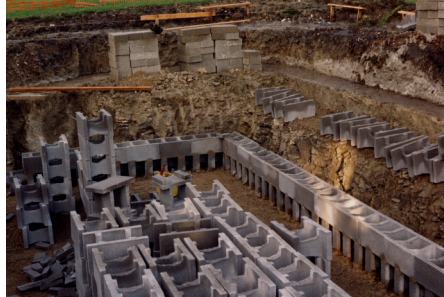
Building blocks continued and horizontal and vertical reinforcing rods introduced to engineer's specifications.
