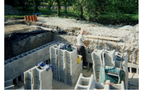
Building blocks continued and horizontal and vertical reinforcing rods introduced to engineer's specifications.
