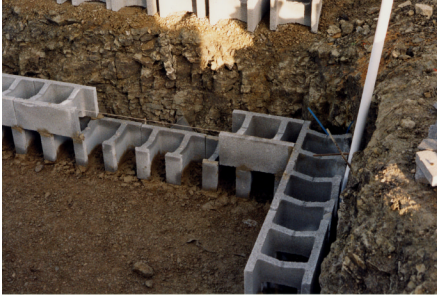
First row of blocks laid to exact measurements and levels.
