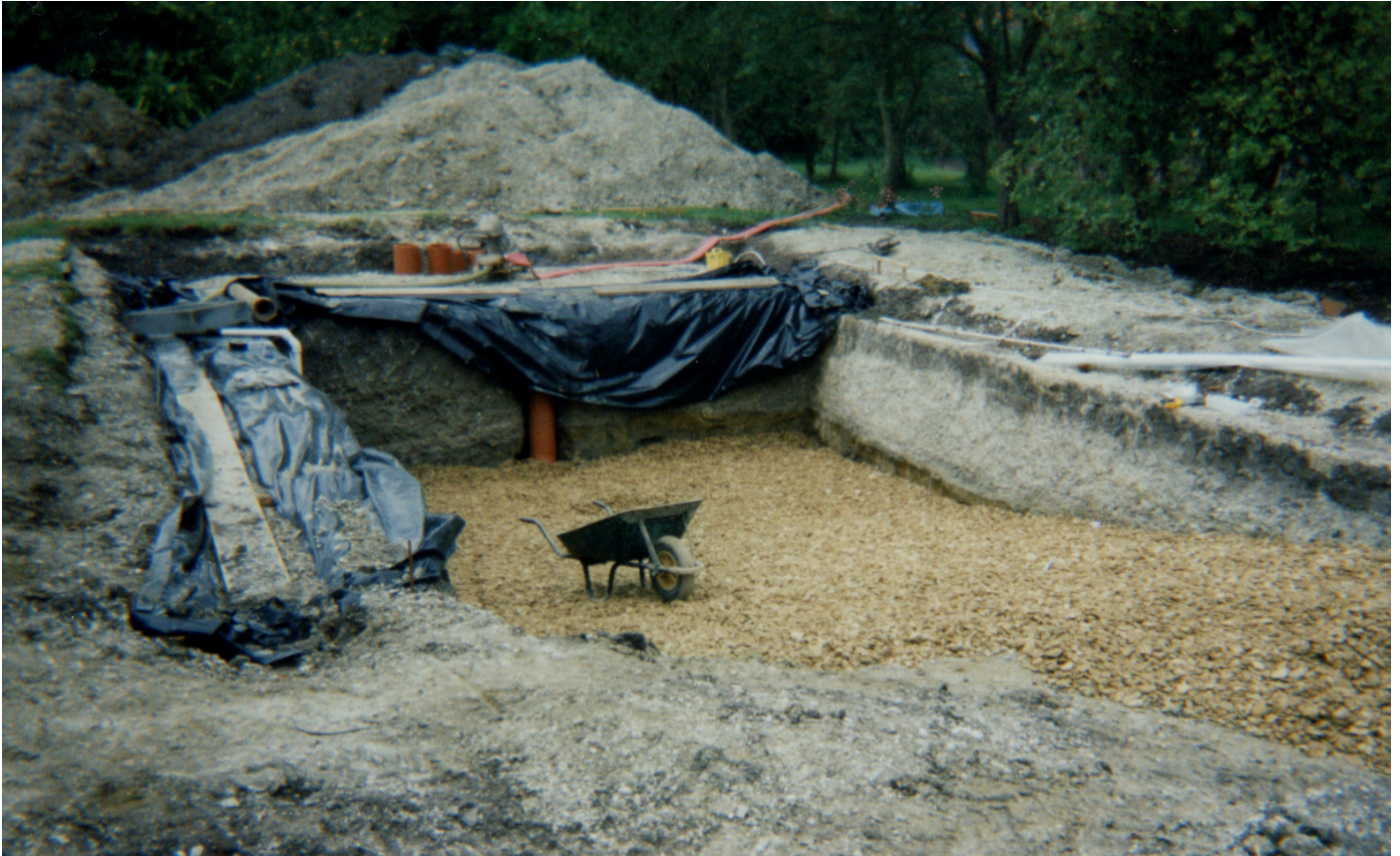
75mm deep-gravel for drainage. Drainage pipe in position
