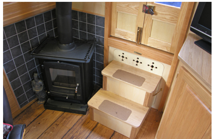
The Portway stove has an inbuilt hearth, side convection fins and a double insulated flue.
