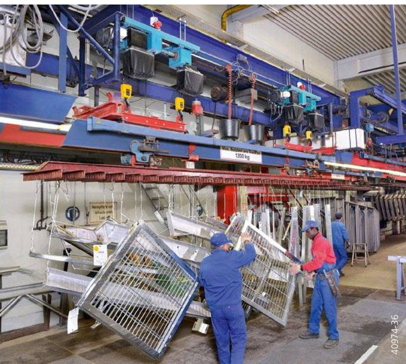
Double chain hoists operating in tandem for handling spreader bars
