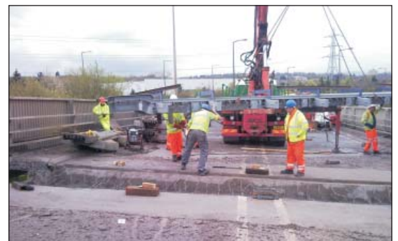
Multi element joint carefully being lifted into the concrete rebate
