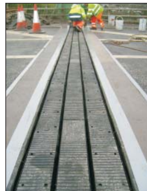
A30 Avers to Tolvaddon Installation of 50 meters TF650 joint.
