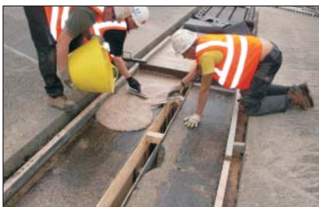
M74 - Port Eglington Viaduct - Glasgow Installation of TF1300 expansion joints.
