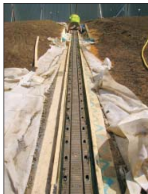
Arundel Square - London Installation of 100 linear meters of TF150 joint.
