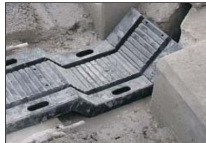
Curb with vulcanised corner joint
