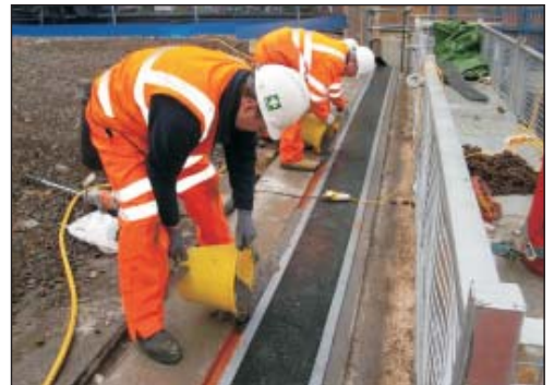
Nosing mortars being poured once joint is fitted in position
