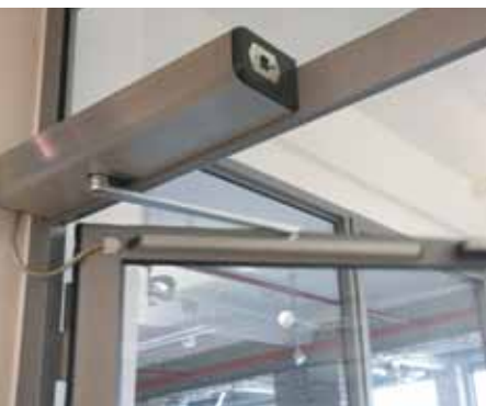
DFA 127 swing door operator with sliding arm
