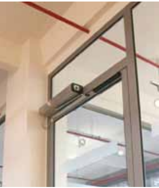
Universal swing door operator DFA 127
