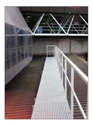
All walkways are built to British Standard BS 5395-1. Fibreglass has a high weight to strength ratio but is lightweight meaning the weight of the walkway does not have to be taken into account when making calculations.
