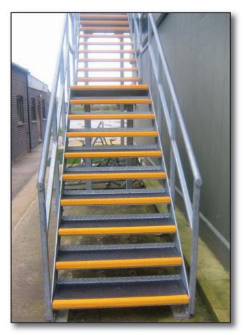
Anti-Slip Tread Covers are a simple and cost effective method of providing an almost instant antislip surface to any stairway whatever the condition of the stairs. Tread covers are extremely durable as a result of a hard wearing quartz grit surface. They have a contrasting nosing for greater visibility and can be cut to any size free of charge.
