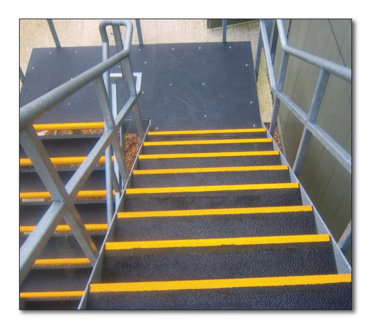
Large sheets of gritted plate are available for landing areas etc. Tread covers conform to BS7976-2 2002 slip resistance test. Our tread covers and plate have achieved a rating considered to be 'better than excellent'.
