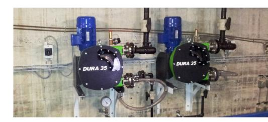
Verder UK recommended a Verderflex Dura 35 peristaltic pump. The Verderflex Dura brand is well established in the water and wastewater industry for the delivery of abrasive and corrosive solutions such as lime chemical, sodium hypochlorite and sodium hydroxide.
