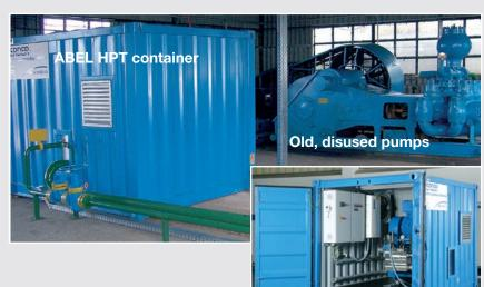
Wiring between the electrical consumers and the control or the frequency converter is not required. This is all already installed inside the container.
