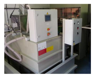
Verder supplied a full temporary dosing solution to allow the chemical room to be renovated with 6 dosing cabinet systems for polyelectrolyte, sodium hydroxide and ferric dosing, a poly makeup tank, control panels and pipework. The entire plant room was repainted, including the floor.
