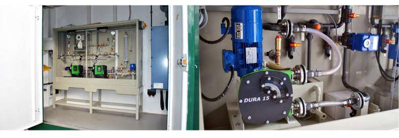
Verder package plant systems are assembled and tested at the Verder Service Centre before being shipped to site for installation, further testing and commissioning.
