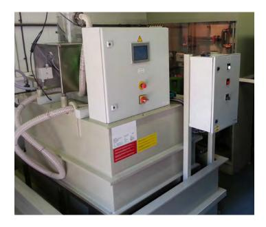
Verder supplied a full temporary dosing solution to allow the chemical room to be renovated with 6 dosing cabinet systems for polyelectrolyte, sodium hydroxide and ferric dosing, a poly make-up tank, control panels and pipework. The entire plant room was repainted, including the floor.
