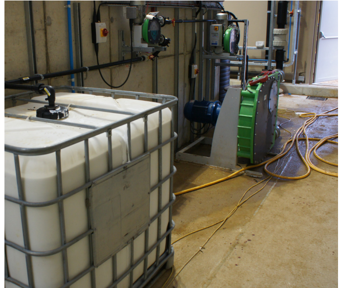
A Verderflex Dura unit dosing a pH buffer into the main tank holding organic matter
